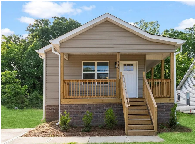
A recently built 1,080 sf home in the City of York
