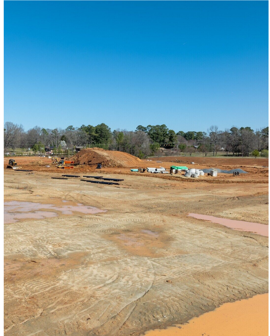
Construction in Rock Hill
