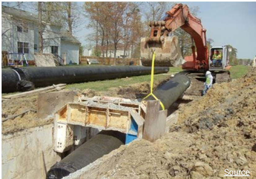
York County stormwater infrastructure construction
